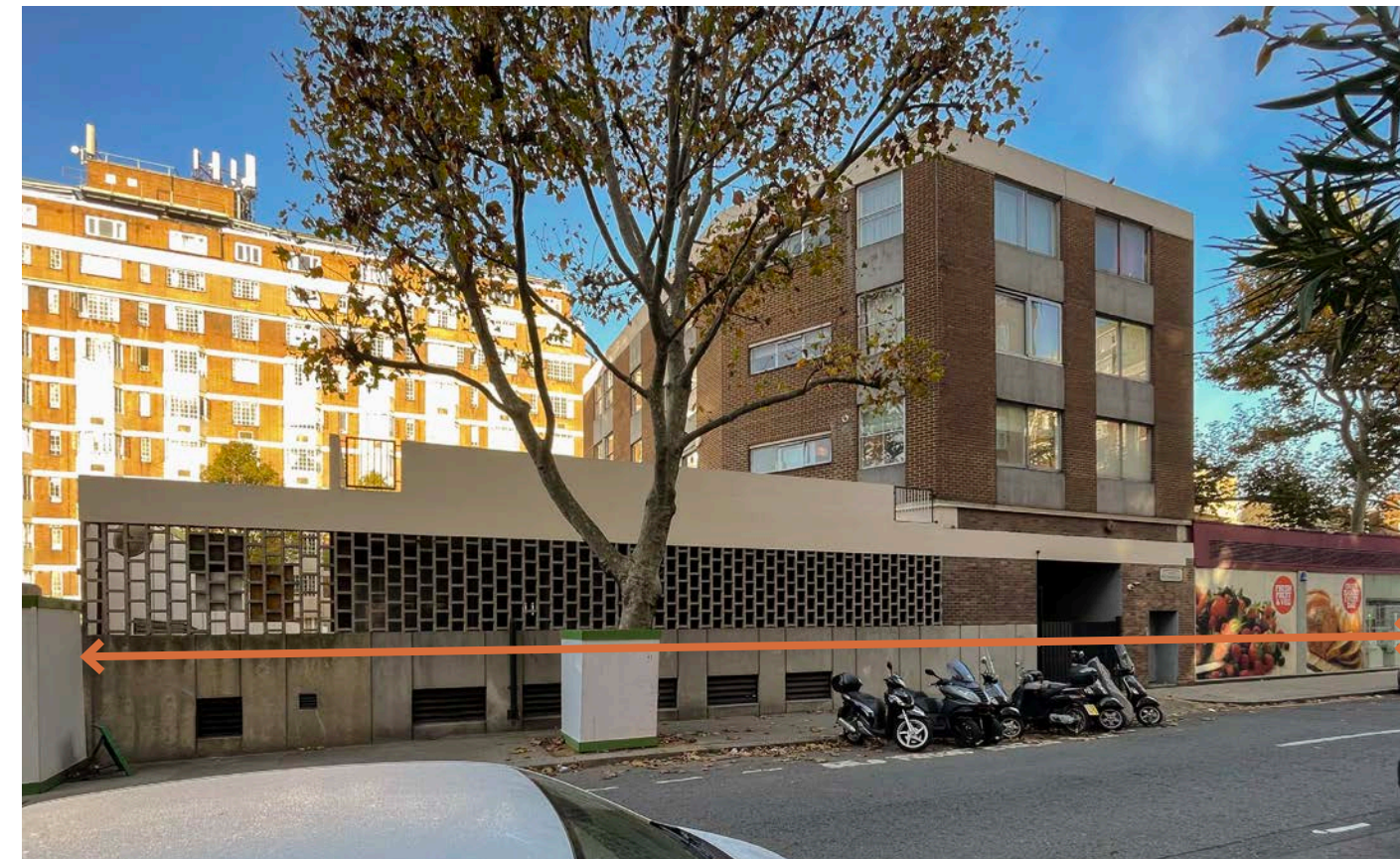
Fig. 5.7.3 - Existing frontage onto Petyward is expanse of blank wall, ventilation louvres and car park screen
