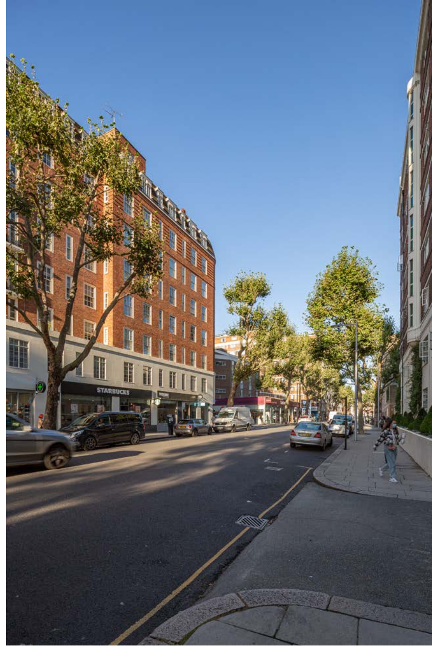
Fig. 5.1.1- Existing and Proposed view towardsThe Site along Sloane Avenue
