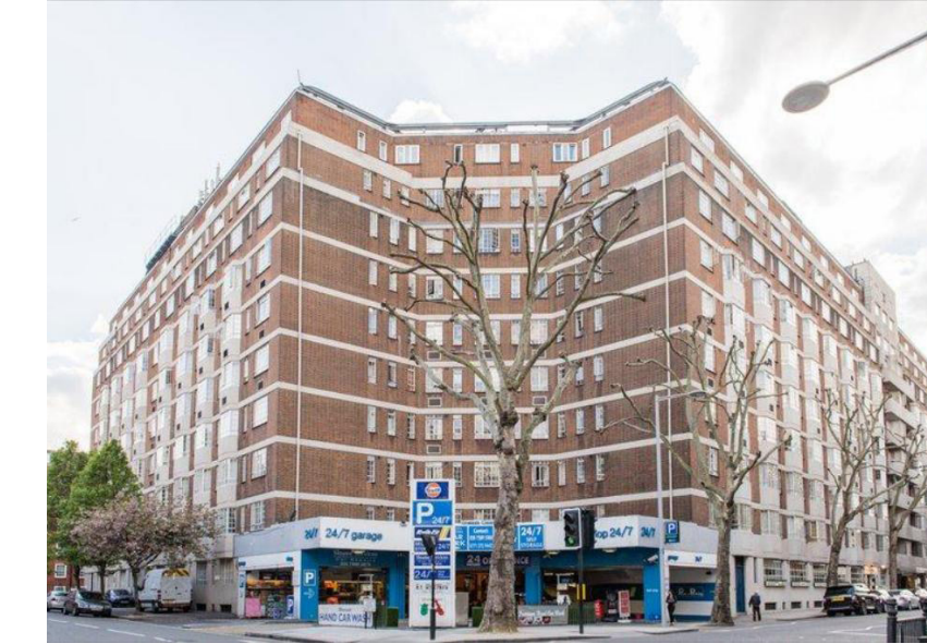
Fig. 2.7.4 - Area 1 - 2 - Chelsea Cloisters
