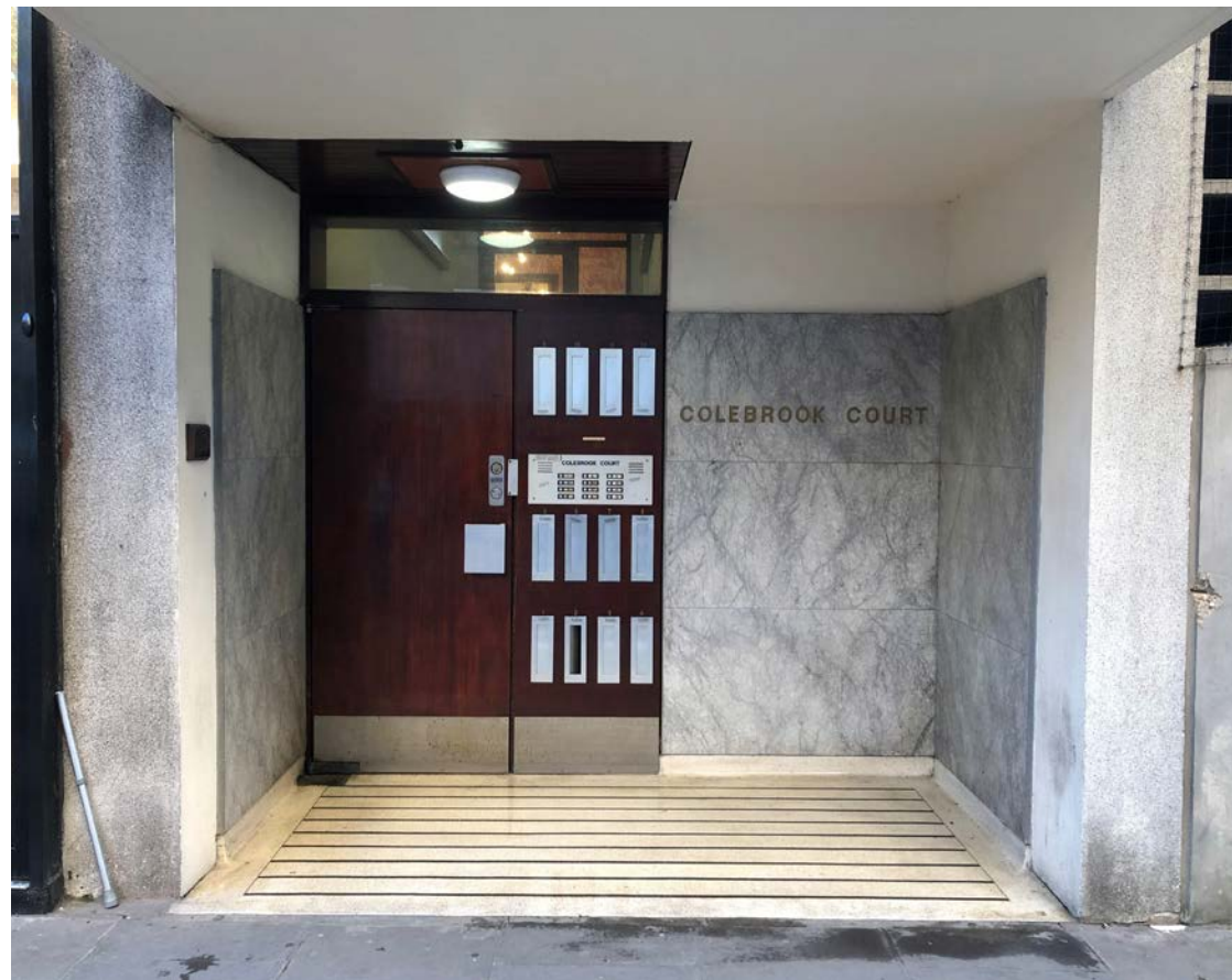
View 4 - View of residential entrance to Colebrook Court
