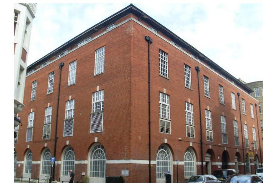
Fig. 2.7.9 - Area 5 - 7 - Telephone Exchange
