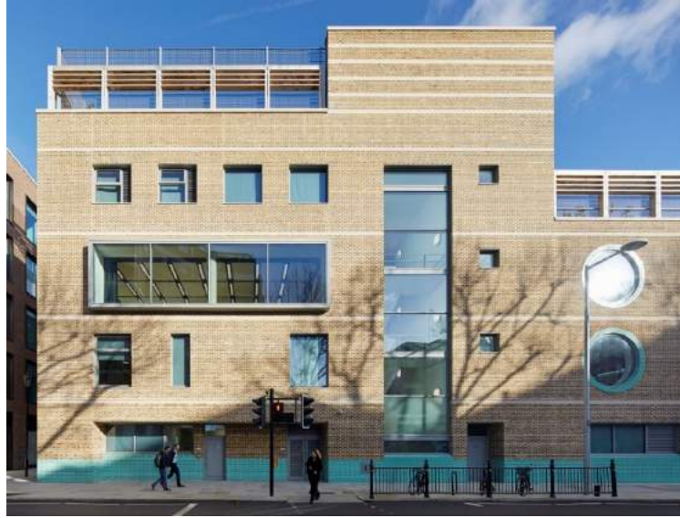
2. New Marlborough School, Draycott Avenue
