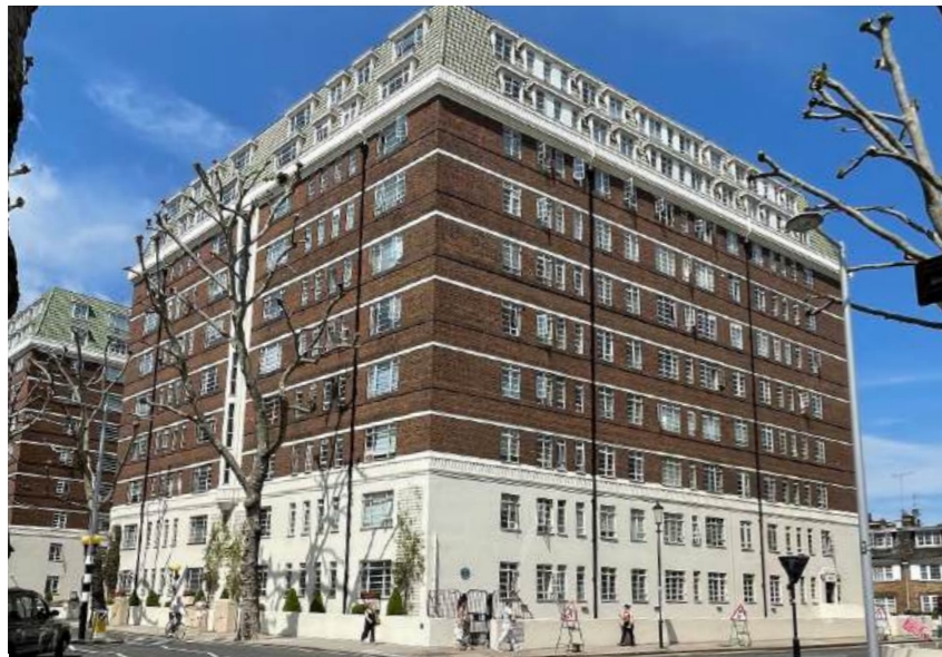
View 1 - View North on Sloane Avenue (Neil Gwynn House)
