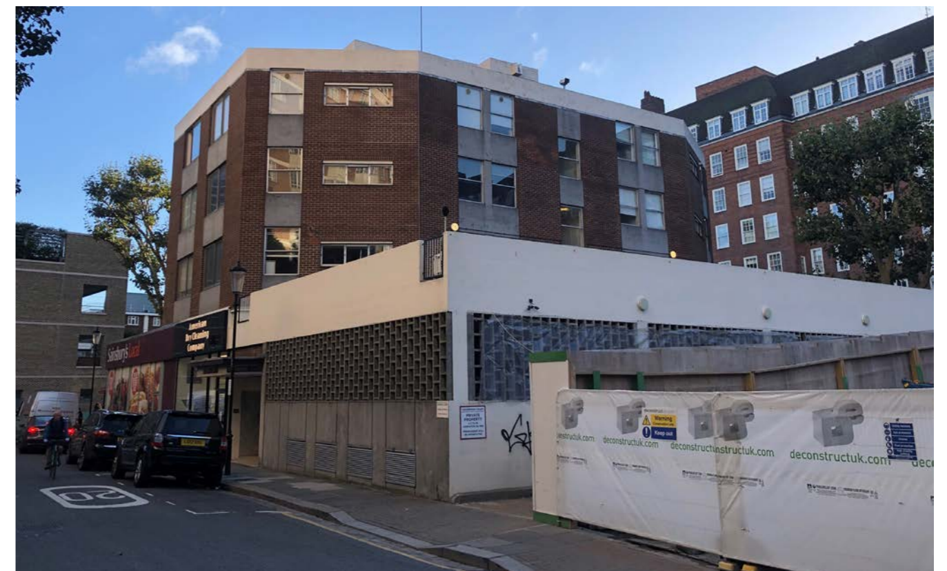
View 3 - Looking towards the residential entrance / rear of Colebrook Court from Makin Street
