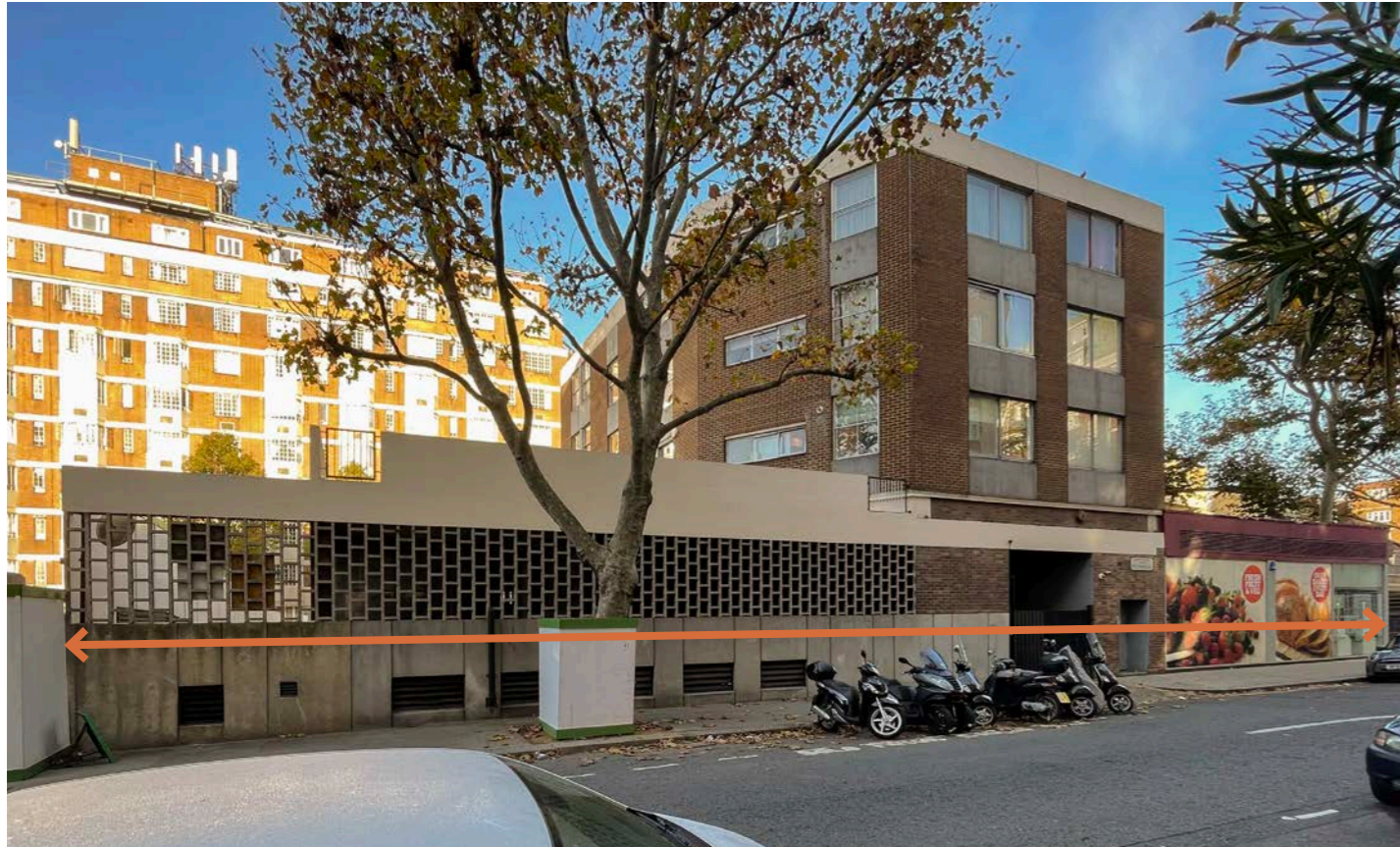
Fig. 5.7.4 - Existing frontage onto Petyward is expanse of blank wall, ventilation louvres and car park screen
