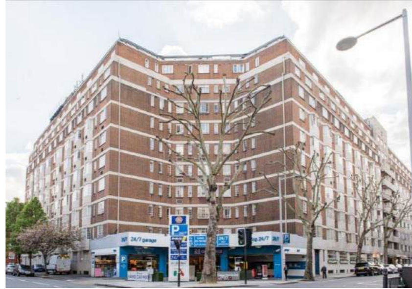
Fig. 2.7.4 - Area 1 - 2 - Chelsea Cloisters
