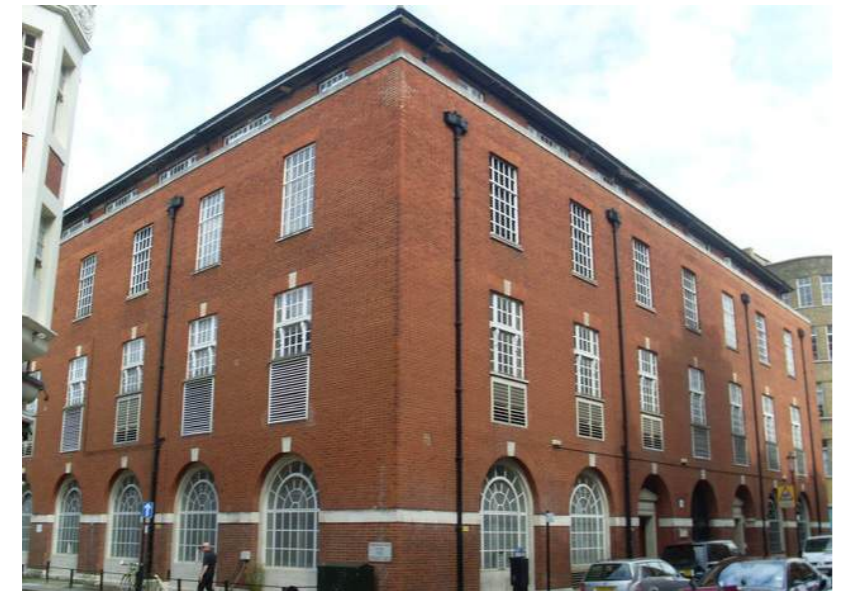
Fig. 2.7.9 - Area 5 - 7 - Telephone Exchange
