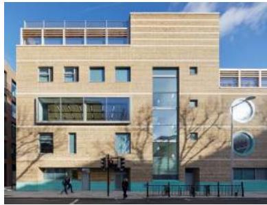
2. New Marlborough School, Draycott Avenue
