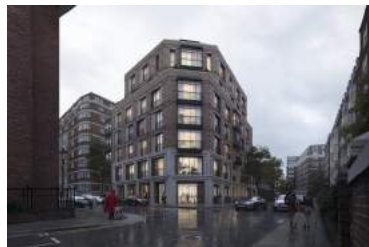
3. No. 2 Lucan Place. Granted, Construction underway
