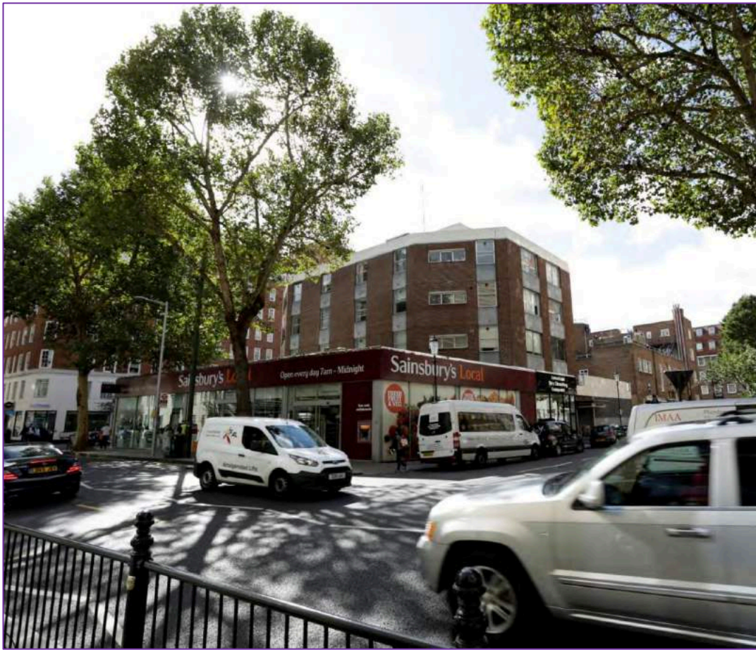
View of existing site from Sloane Avenue
